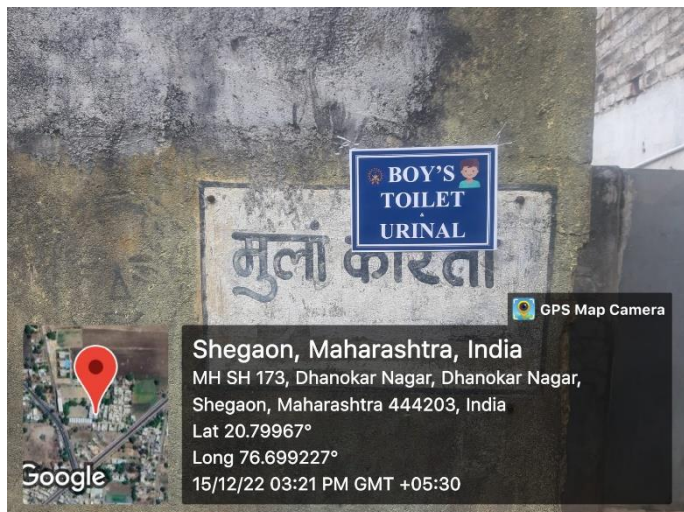
Boys Toilet Urinal
